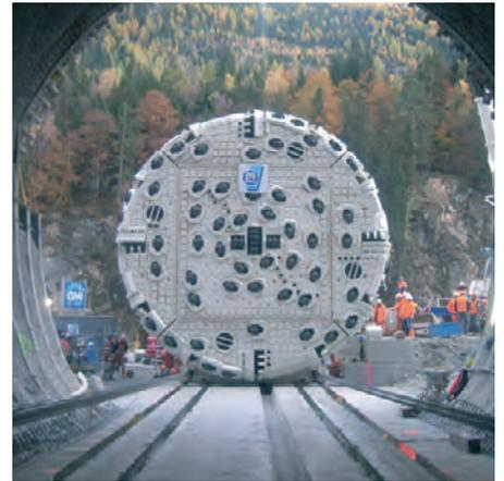
Tunnelbohrmaschine Nant de Drance.
